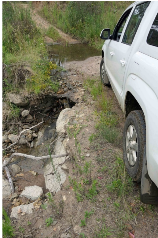
Figure 13: Road damage done in a 2020 post-fire rainstorm.
