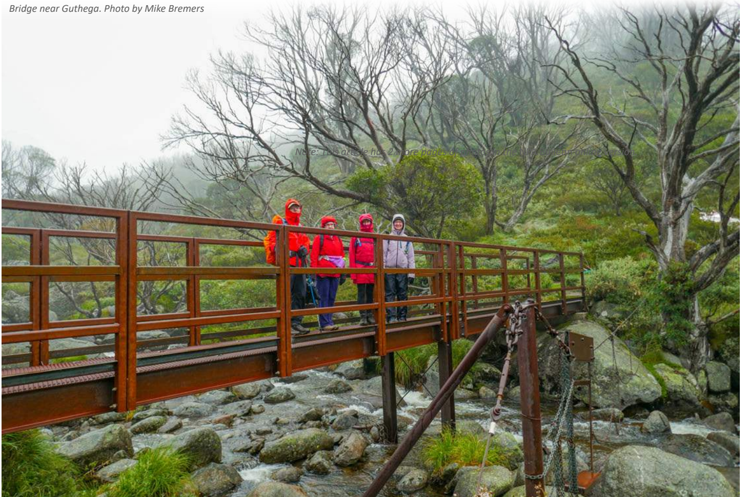
Bridge near Guthega. Photo by Mike Bremers
