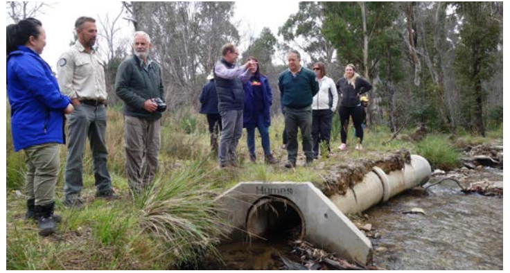
Washed-away culvert at Bimberi Creek. Photo by Allan Sharp
