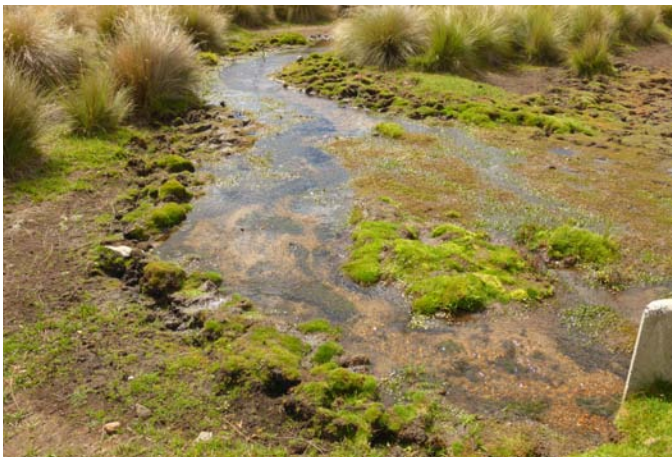
Culvert at fire trail junction, Seventeen Flat. Photo by Di Thompson.
