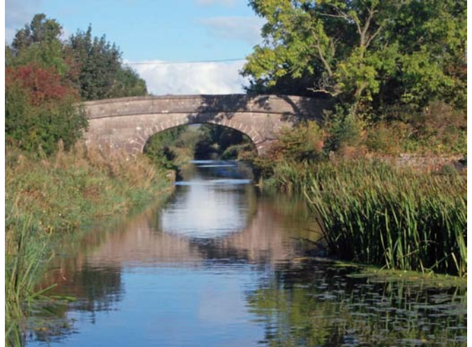
A bridge over the Lancaster Canal. Photo by Tim Walsh.
