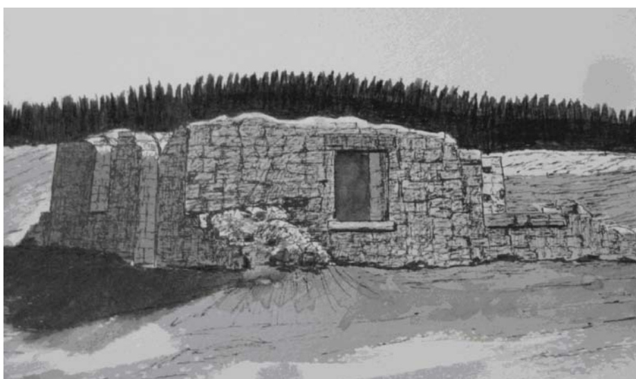
Ink and ink wash sketch of Colliers Homestead ruins by Gary Thompson, 2014. The mortar capping laid by ranger Dean Darcy and members of The Friends, can be seen clearly on the tops of the walls,
