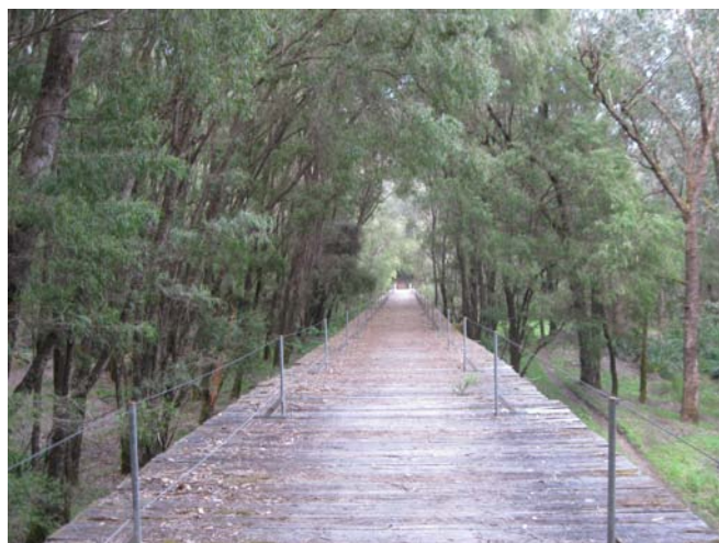
Old trestle bridge Photos Judith Webster
