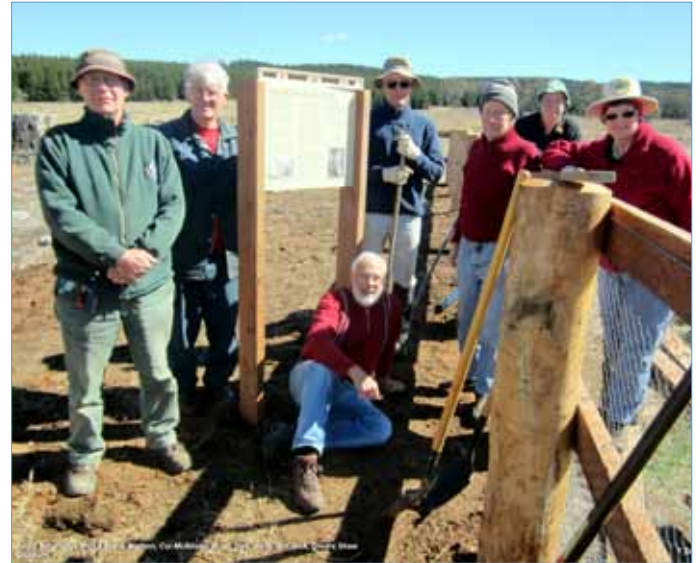
Work party at the recently erected interpretive sign at Glenburn Homestead, September 2012. Photo Max Lawrence.
