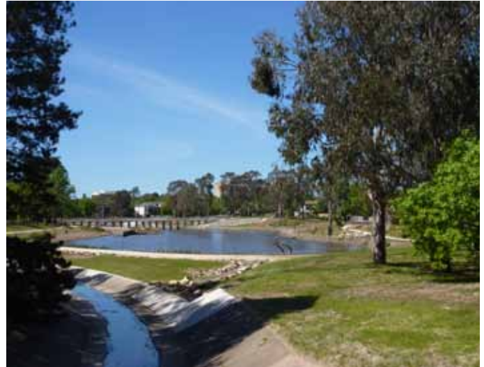
The new Lyneham Wetland.
