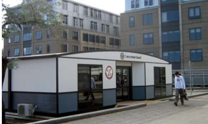
'The office'. Formerly a construction site office, in 2010 the building is occupied by NPA and ConsACT. Photo Max Lawrence
