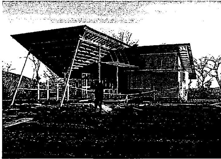
Mt Franklin chalet replacement during construction, 26 May 2007. Photo Michael Goonrey
