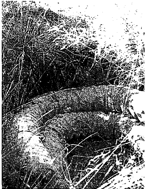
"Coconut logs" wedged into an eroding corner of the creek. Photo Martin Chalk
