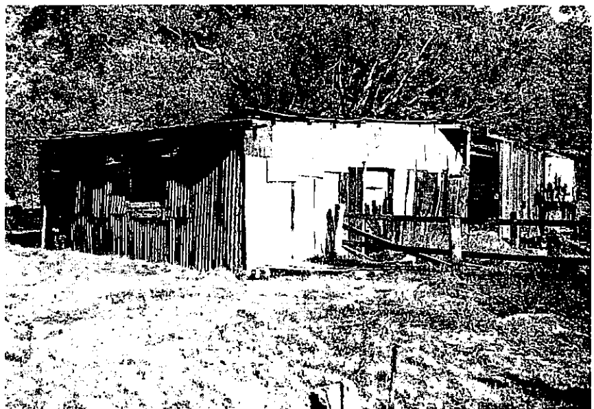
The front wall of the woolshed showing the gable end of the original small shed. Photo taken in 1994 by Babette Scougall
