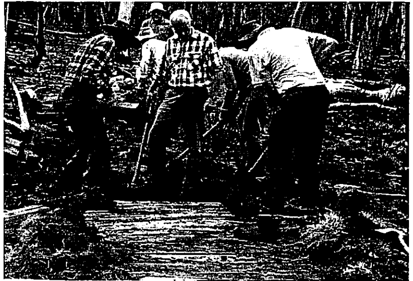
Above. Laying the corduroy track (l to r) Frank Clements, Phil Gatenby, Allen Bills.
