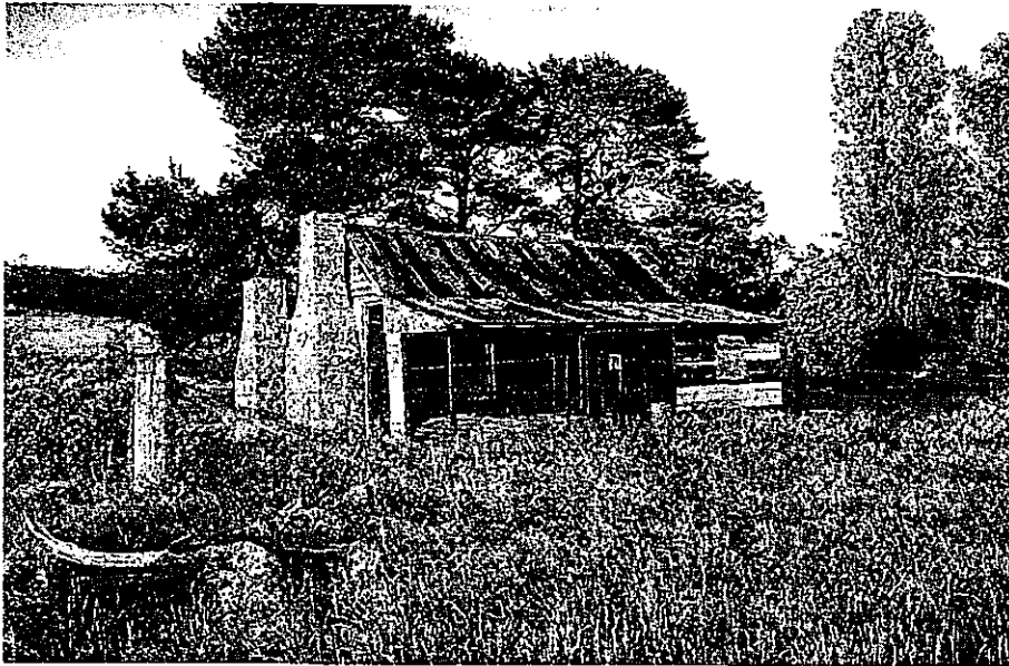
Westerman's Homestead at dawn, December 1998, showing newly restored chimneys. Photo Martin Chalk.
