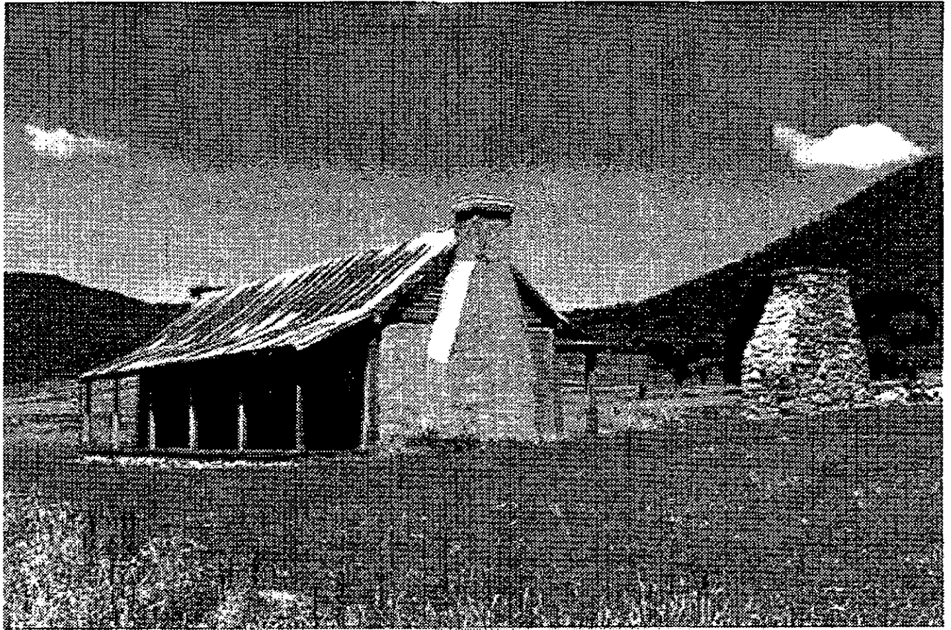
Orroral Homestead after the restoration. Note the restored stone kitchen chimney and the replaced gable timbers and replastered chimney on the homestead itself. Photo by Graeme Wicks
