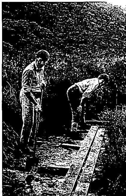
Below: Making a plank track in the Budawang.
