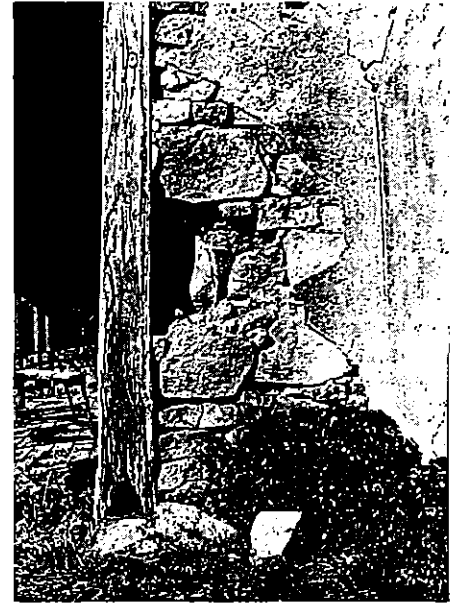
Rotten cornerpost and collapsing masonry, Orroral Homestead.
