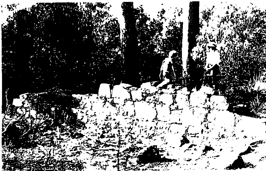
The western wall of the Bittangabee Bay ruins. The rough dressing of the stone in comparison to the fine stonework of the Boyd buildings is very evident. This section is the highest point the walls reached before construction was abandoned.
