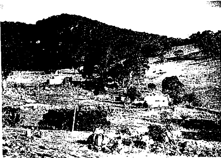
GLENDALE HOMESTEAD — Demolished and a maintenance depot erected near the site.
