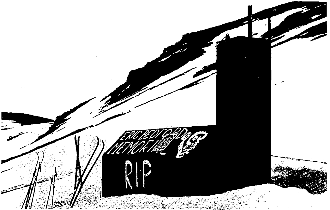
The emergency hut, with its message, erected at Lake Albina to replace the now demolished larger Albina hut.
